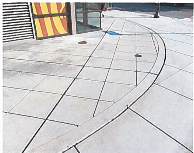
Concrete Paving with Score Joints (or similar)
