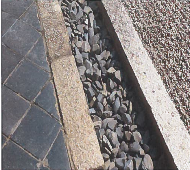
In-Pavement "Runnel" (or similar)
