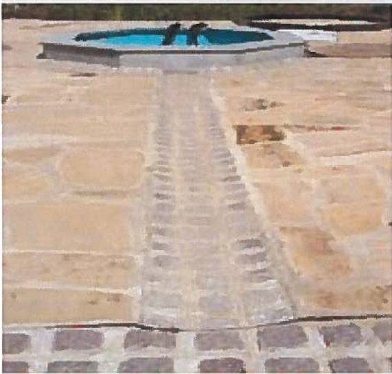
Cobbles sloped to form runnel
