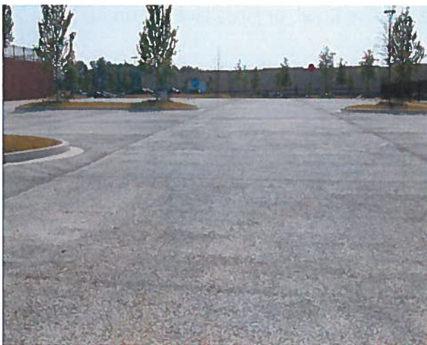
Pervious Concrete Paving (or similar)
