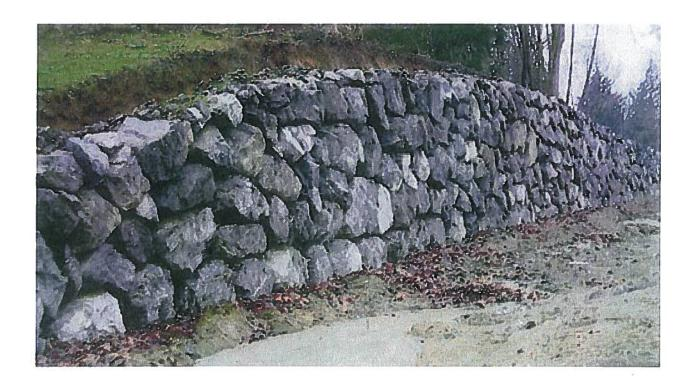
This is an example of a typical rockery retaining wall, similar to what would be used at the AutoZone project.
