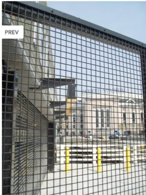
Sample of two different types of grating over garage openings
