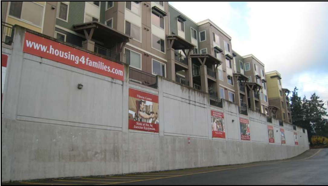
Example of scale of concrete wall on south side
