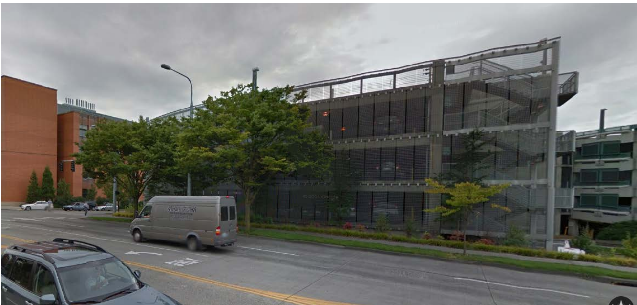
This is the photo of a garage that uses a similar metal screen system to the one that the applicant has proposed. Landscaping in this photo helps soften the façade.
