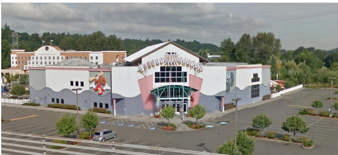
Figure 3. View from SW Grady Way looking northwest
