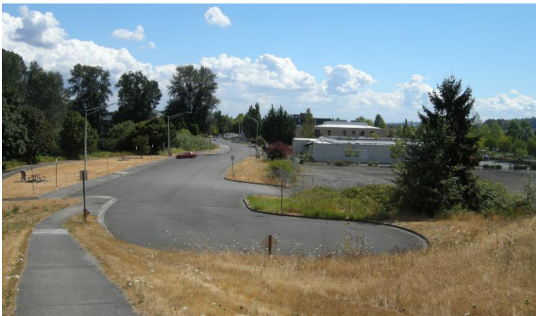
Figure 4. Existing conditions—looking south from Tukwila Pkwy (Green River Trail, Christensen Road, and project site)
