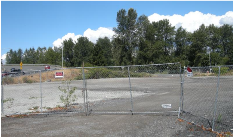
Figure 3. Existing Conditions—project site looking NE from Andover Park E.
