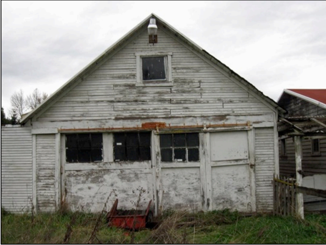
Figure 9. Barn/stable front elevation; view to the south.
