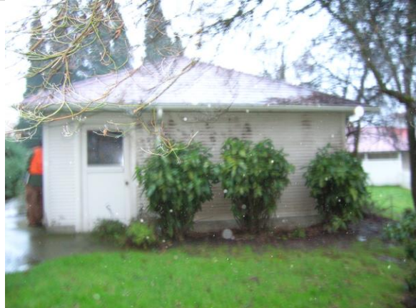
North Elevation-Garage-Looking South North Elevation-Garage
