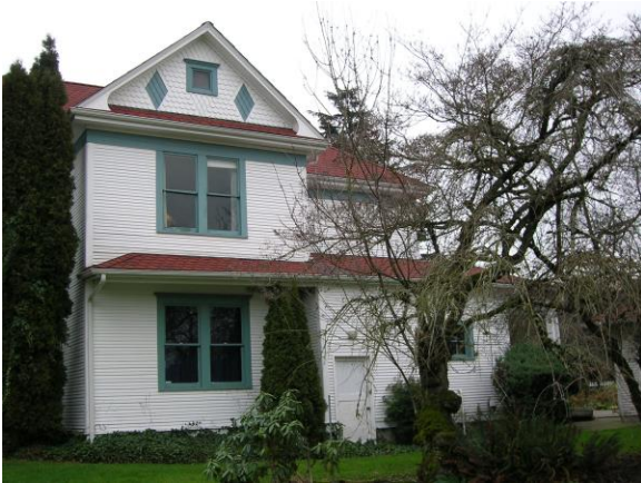
Right 2/3 west elevation looking east Right 2/3 West Elevation
