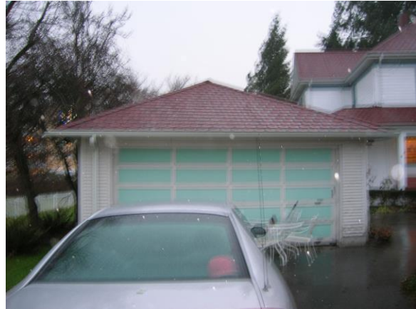
South Elevation-Front-Garage-Looking north South Elevation-Front-Garage
