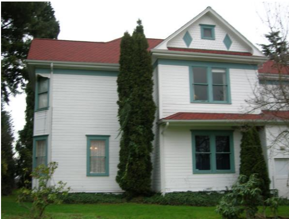
Left 2/3 west elevation looking east Left 2/3 West Elevation
