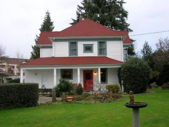
South elevation looking north South Elevation
