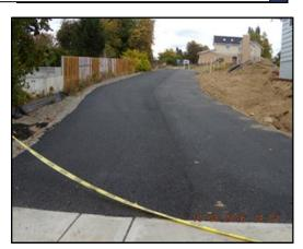
Asphalt paving half pervious half impervious
