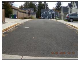
Access street using pervious material
