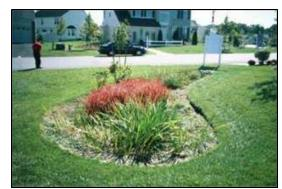
Residential scale bioretention facility. Catch basin in place to drain overflow.
