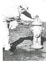
10. Replace bonnet. Turn operating nut in closing direction to engage stem. If bonnet has filler plug, make sure that the filler plug hole is aligned with the offset portion of the oil reservoir. Bolt in place.
