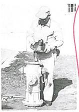
2. Remove four bolts in stuffing box. Lubricate A-24099 Brass Sleeve. Slide Sleeve over threaded area of stem to protect "O" rings from damage by threads, Lift stuffing box off carefully. Remove brass sleeve.
