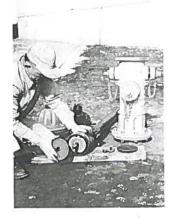
5. Remove lower stem nuts while stem and valve assembly is still in seat wrench. Replace damaged or worn parts.
