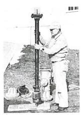
7. Loosen seat wrench extension (or operating nut) so seat ring has some float in seat wrench. Replace complete working parts and seat wrench assembly in hydrant barrel.
