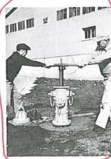
gages lugs on seat ring. Screw seat wrench stem extension on a unit from hydrant barrel. " to hydrant stem until pin engages top of seat wrench. (If non-adjustable type, use operating nut instead of seat wrench stem extension.) Shut off water at the gate valve. Turn wrench counter-clockwise to unscrew seat ring.
