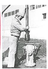
4. Lift stem, complete valve mechanism, and seat wrench as
