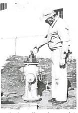
9. Check stuffing box gasket. Lubricate A-24099 Brass Sleeve. Slide Sleeve over threaded area of stem to protect "O" rings from damage by threads. Place stuffing box in position and bolt to barrel. Remove Brass Sleeve. Pour Mueller Hydrant Lubricant into oil reservoir until THREE-QUARTERS of an inch from top:
