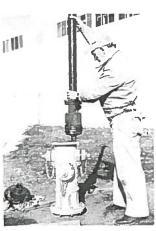
8. Screw seat ring in place by turning seat wrench clockwise. Turn water on at gate valve. Remove seat wrench.
