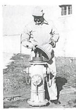
1. Remove four bonnet bolts and turn operating nut in the opening direction until free of the stem. Remove bonnet.
