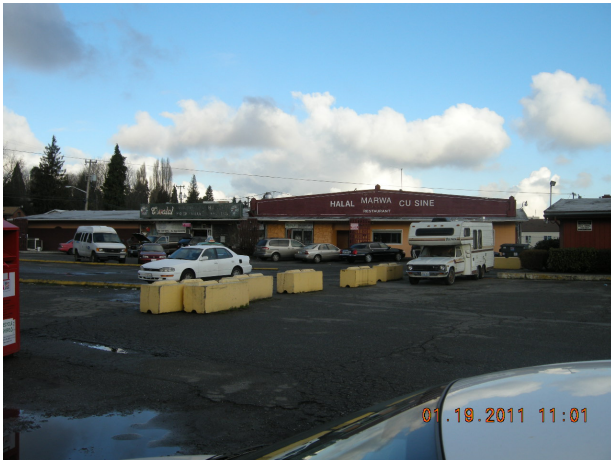
Existing Commercial Building (to remain)
