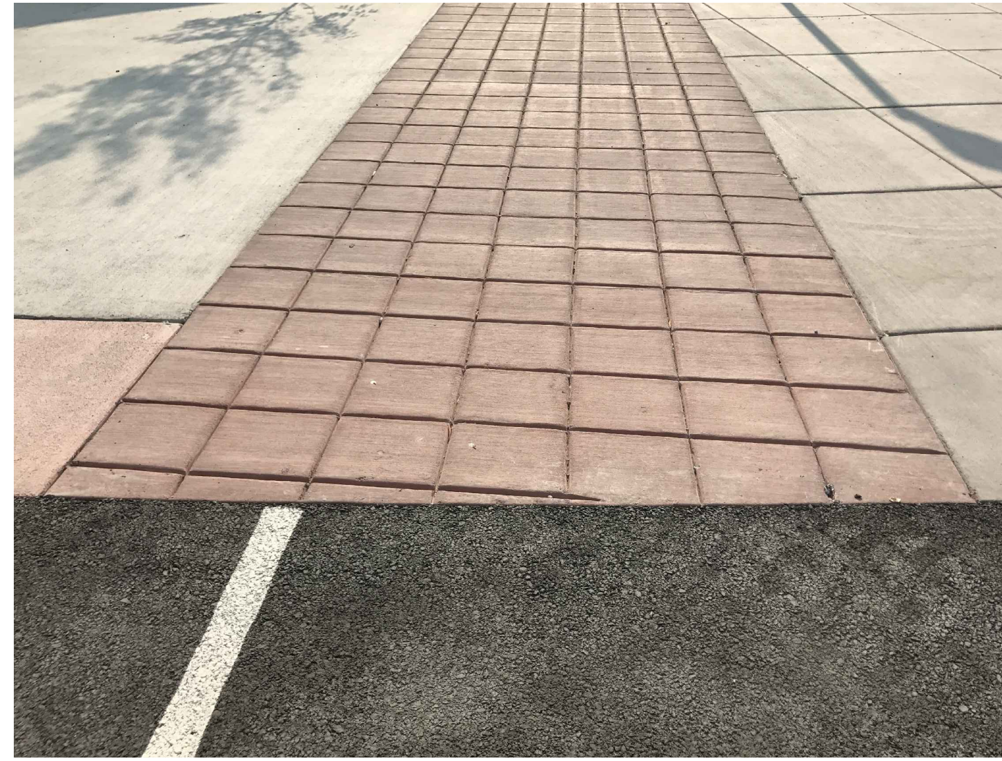
2 COLORED CONCRETE CROSSWALK NOT TO SCALE
