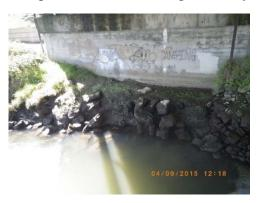
have caused scour damage at the bridge abutments and at the north approach roadway. Because the bridge foundation depths are unknown and there is active scour, the City has implemented a scour Plan of Action (POA) for high flow events. Additionally, existing riprap at Pier 2 is either washing away or is falling into a scour hole developing on the river side of the pier. The bridge is the only access for the BNSF intermodal yard located at the end of South 124<sup>th</sup> Street as other
