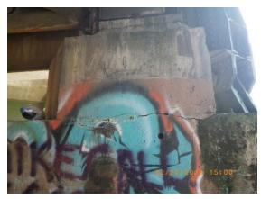
The interface cracking has been documented since 2001 (upper photo) and the cracks are currently opening and starting to spall. In addition, there has been documented evidence for many years of the deterioration of the reinforcing steel as evidenced by rusty leaching. These problems may have been initiated during the April 29, 1965 South Sound Earthquake and were likely compounded by the February 28, 2001 Nisqually earthquake. However, the damage
