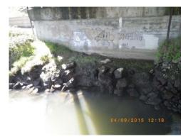
have caused scour damage at the bridge abutments and at the north approach roadway. Because the bridge foundation depths are unknown and there is active scour, the City has implemented a scour Plan of Action (POA) for high flow events. Additionally, existing riprap at Pier 2 is either washing away or is falling into a scour hole developing on the river side of the pier. The bridge is the only access for the BNSF intermodal yard located at the end of South 124<sup>th</sup> Street as other
