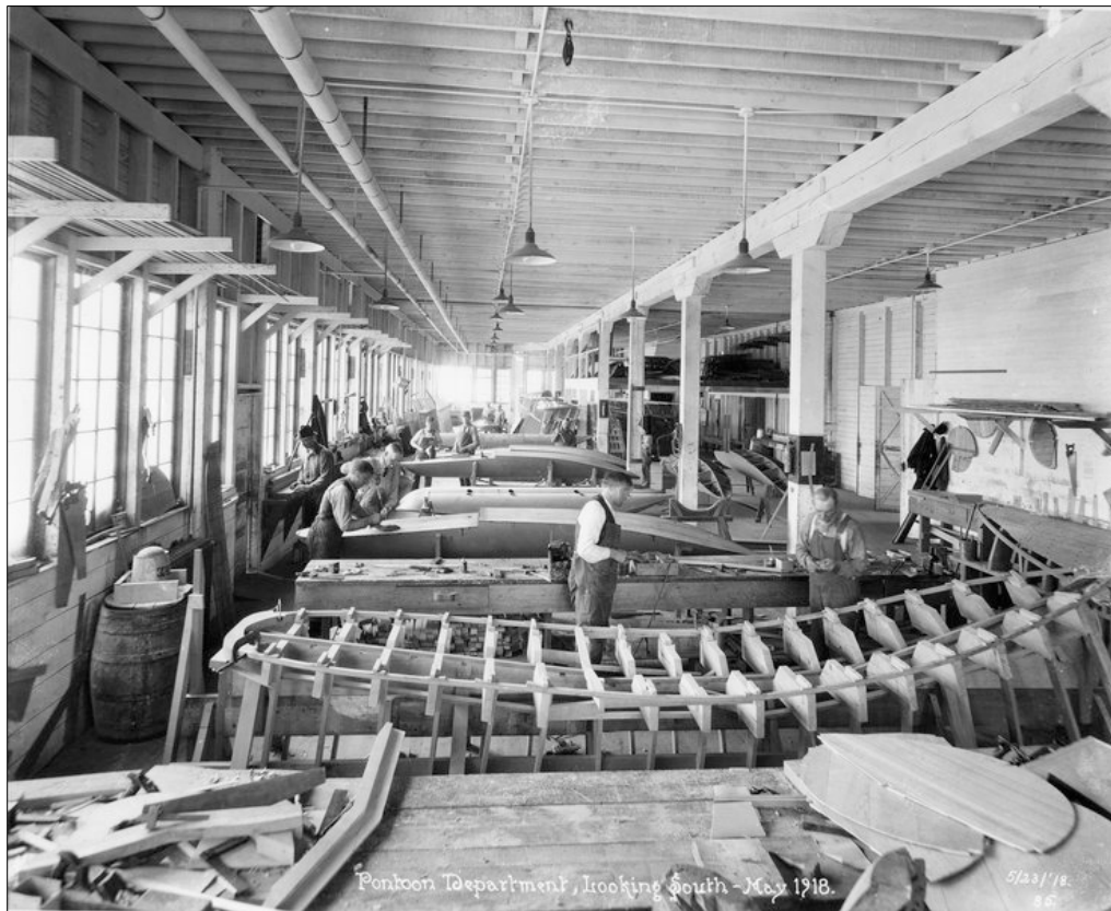
Figure B7. Red Barn, first-floor interior, May 23, 1918. Boeing Co. Archive, P85.
