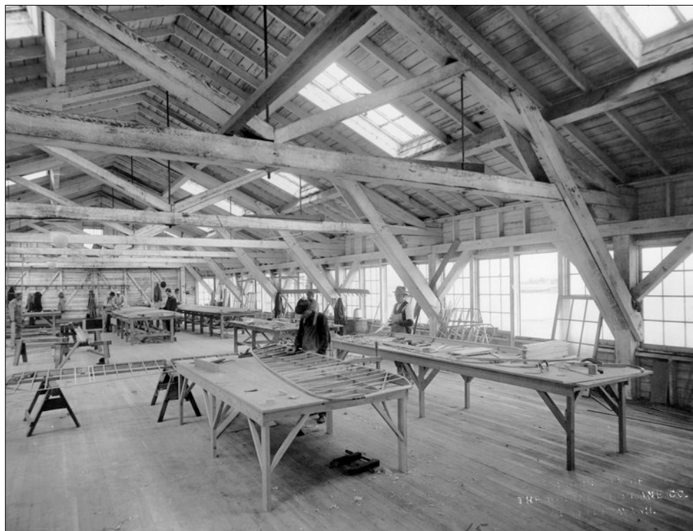
Figure B8. Red Barn, second-floor interior, ca. 1918. Boeing Co. Archive, P15.
