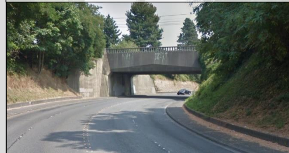
S. Ryan Hill Way at Beacon Avenue S.
