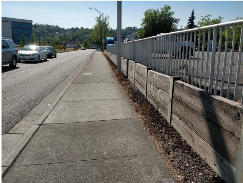
Figure 5. Retaining wall of 1.5’ – 3’ in height along Minkler frontage will be replaced by a 9’ sloped landscaping strip and 6’ wide sidewalk at-grade with the development pad.
