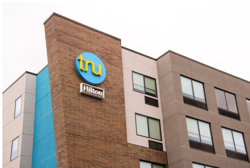
Figure 12. Tru in St. Charles, Missouri featuring brick detail
