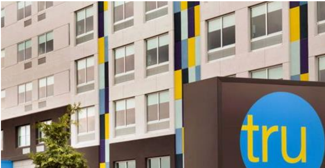
Figure 13. Lancaster, Pennsylvania Tru showing windows slightly inset
