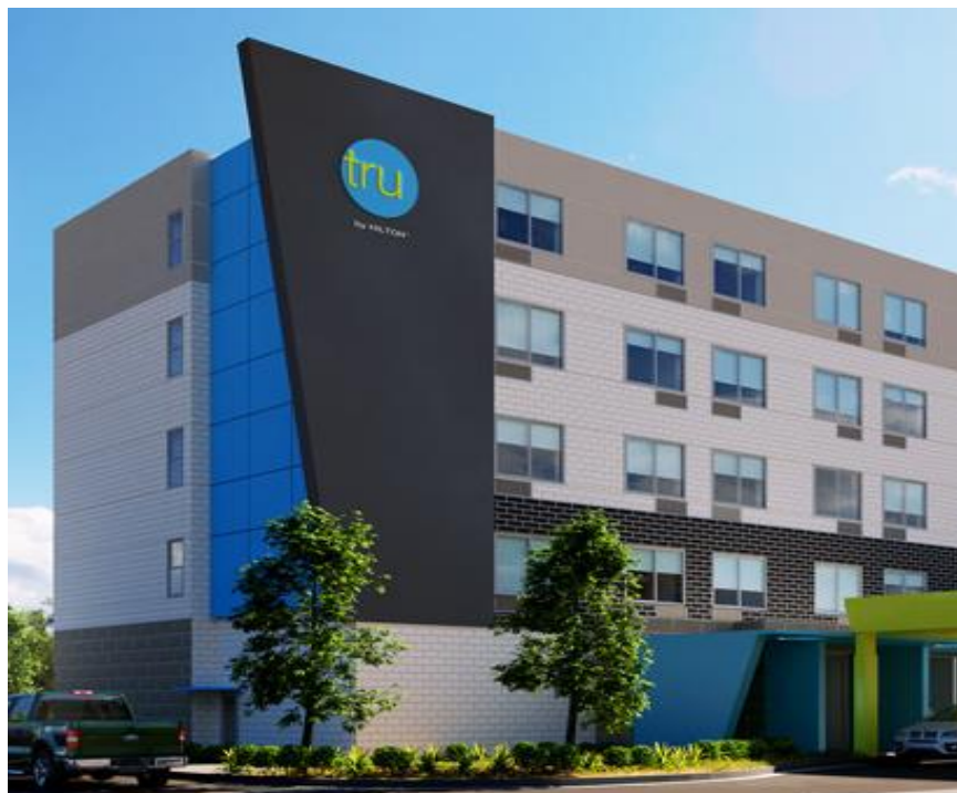
Figure 11. Troy, Michigan Tru hotel, featuring a top floor distinguished from lower floors by material and color
