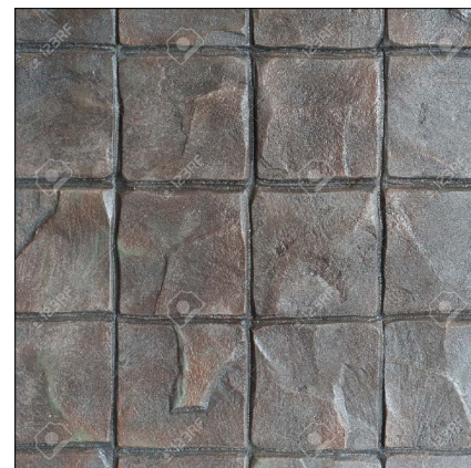
STAMPED CONCRETE VEHICLE AREA - PORTE COCHERE
