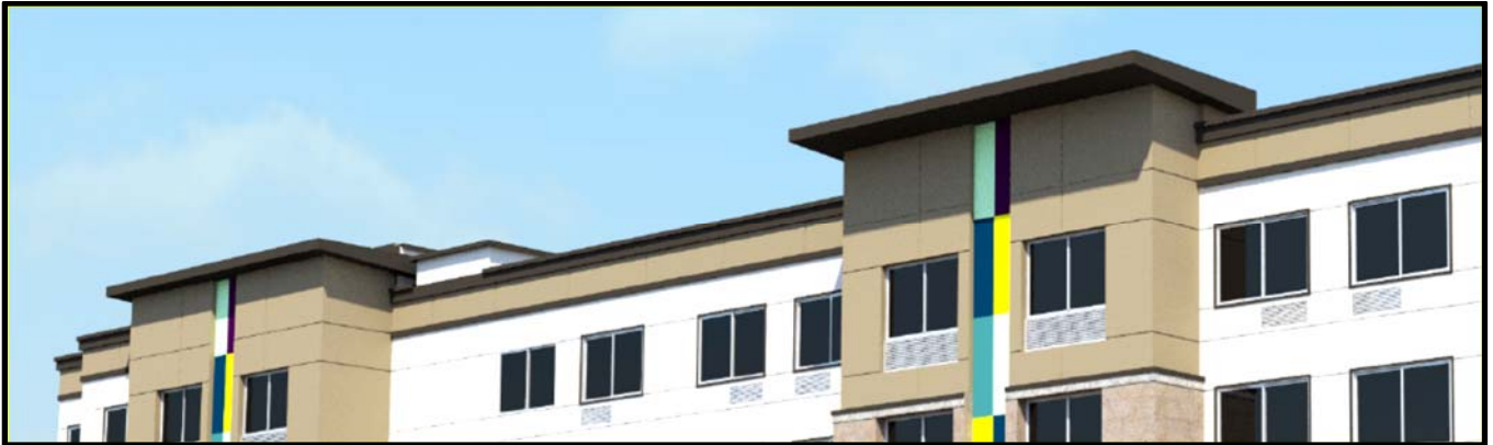
Figure 5. The western façade roofline features projections, molding, and color banding to emphasize the building’s “top”.
