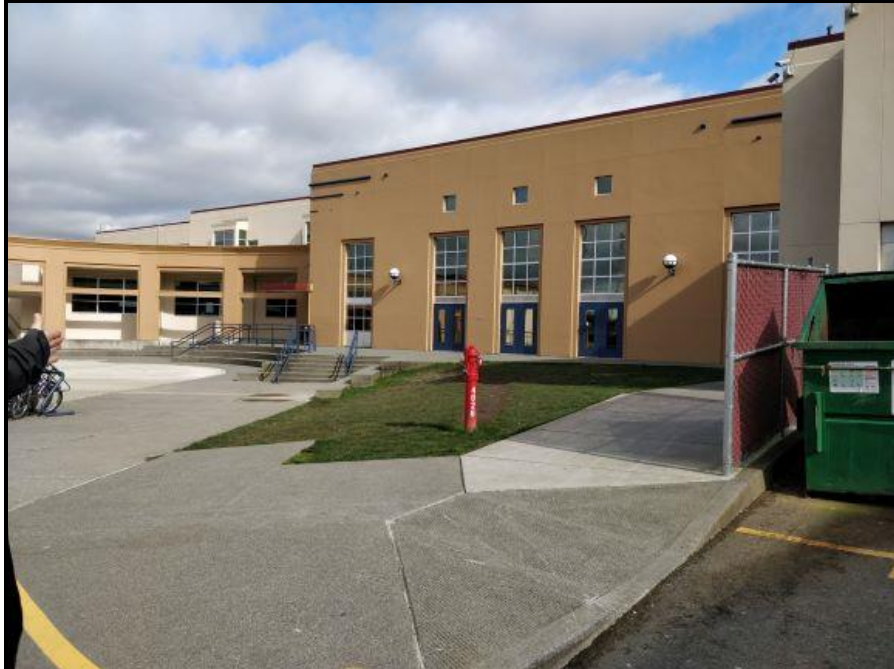
Figure 3. Existing commons/cafeteria west-facing façade and green space
