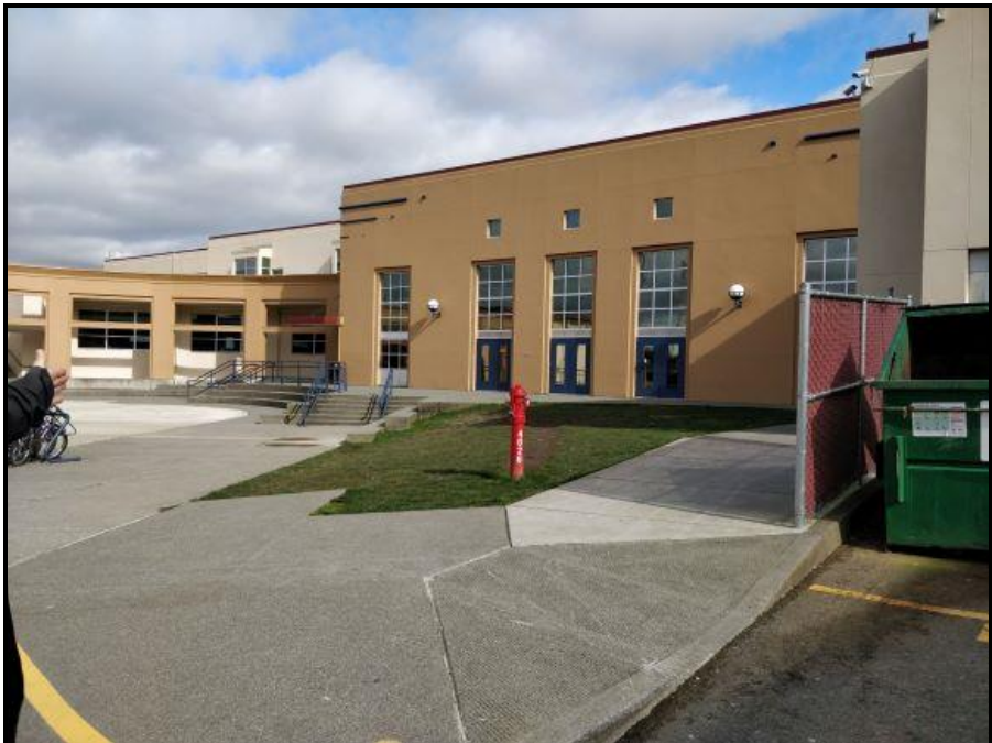
Figure 3. Existing commons/cafeteria west-facing façade and green space
