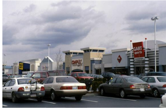
Photo 4. Parkway Super Center
