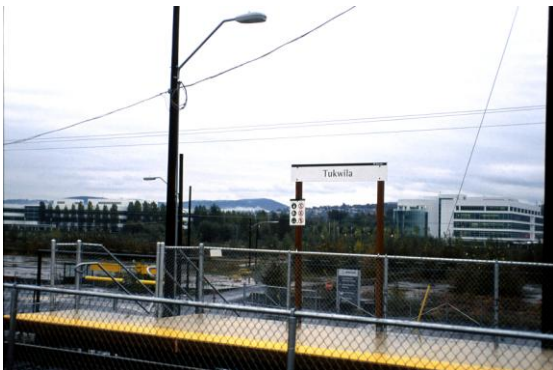
Photo 8. Temporary Tukwila Longacres Station
