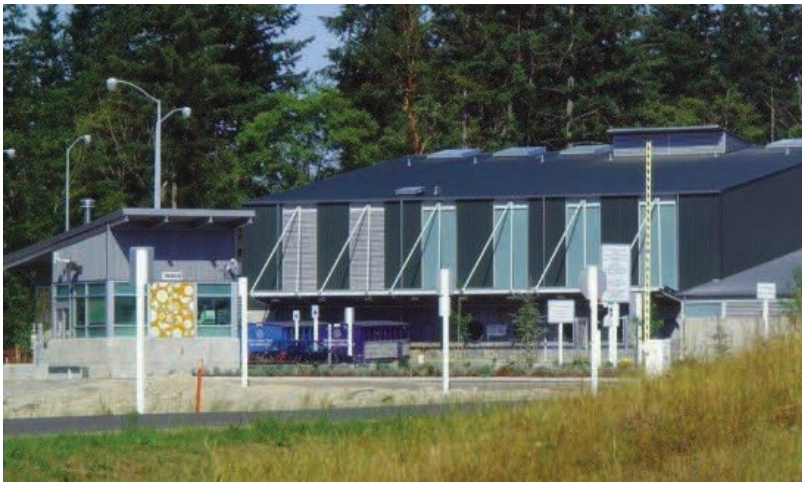
King County Transfer Station
