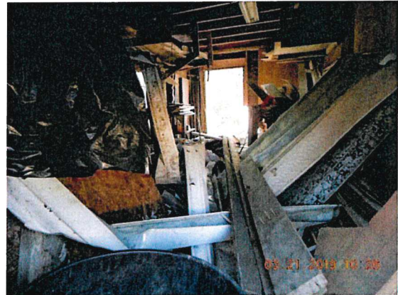
Interior of detached garage
