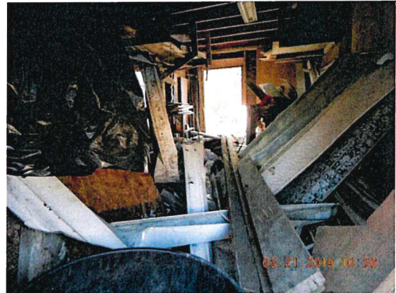
Interior of detached garage
