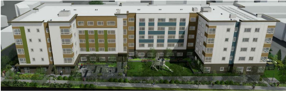
Building Elevation – West Side
