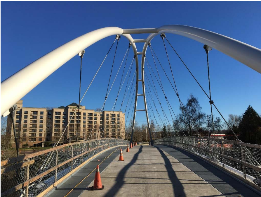
Tukwila Urban Center Pedestrian Bridge
