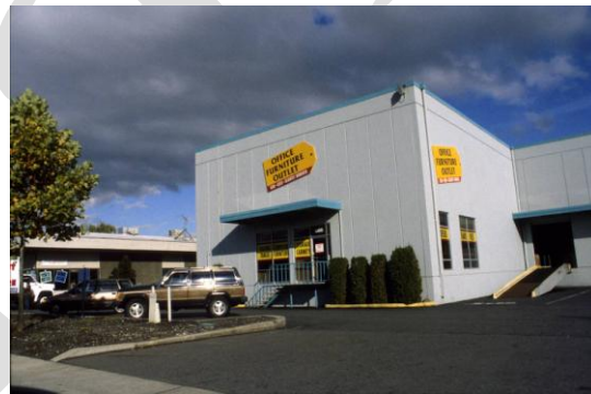
Photo 6. Lower value office & Warehouse
