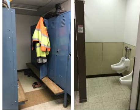
EXPANSION OF MENS RESTROOM AND RELOCATION OF LOCKER ROOM CONSTRUCTION COST - $150,000
