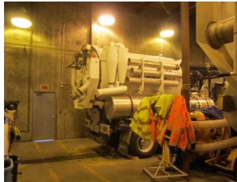
ADDITIONAL STORAGE FOR CREW'S GEAR/ MUD ROOM CONSTRUCTION COST - $60,000
