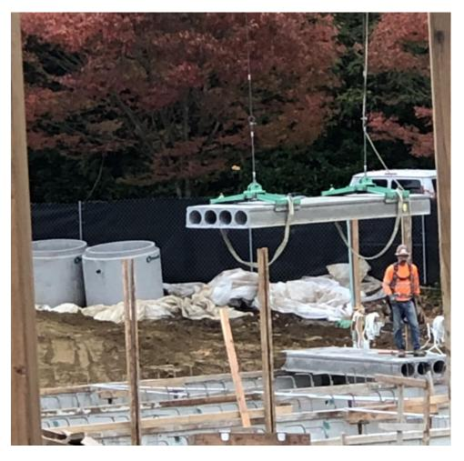
**Detention Vault Hollow Core Metal Planks**
