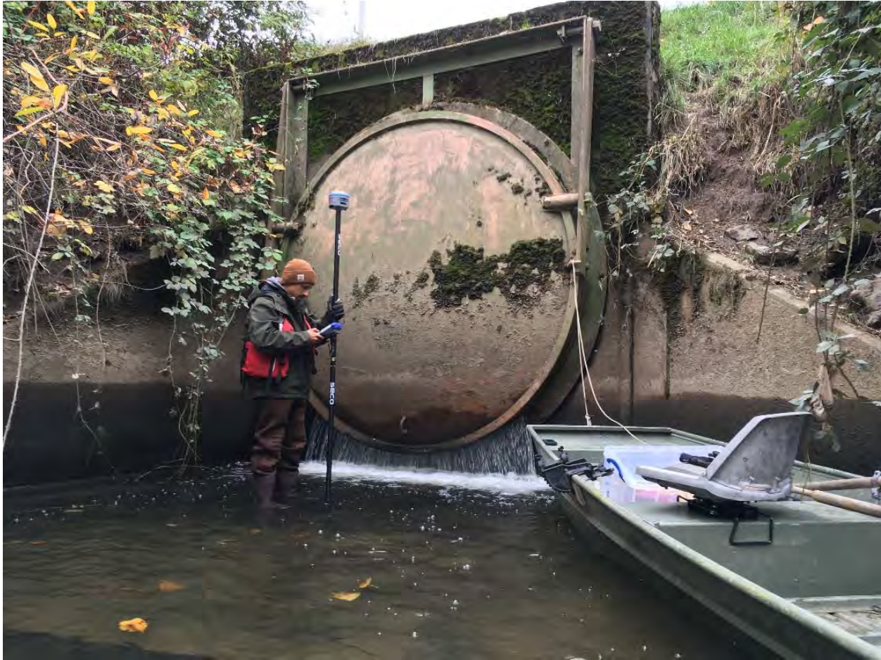
Photo 1. Existing Gilliam Creek flap gate, wing walls, and splash pad.
