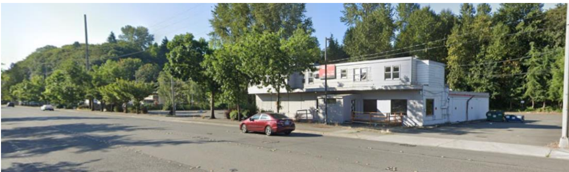
Fig. 4: View of existing development/site looking southeast from Interurban Ave S.
