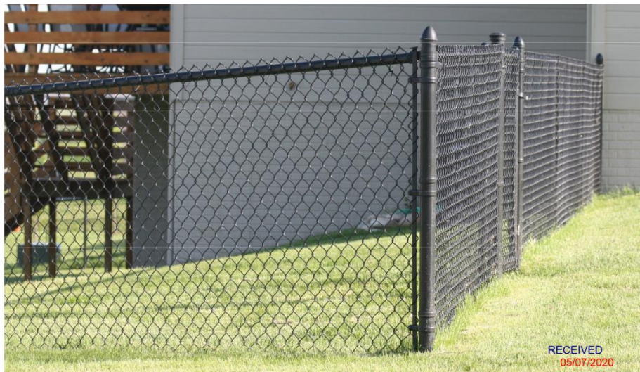
Fig. 9: Chain link fence to be used around service yard. Black vinyl screening to be installed to provide visual screening.
