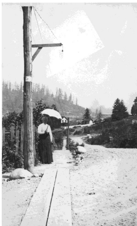
Riverside Avenue and Highland Drive
