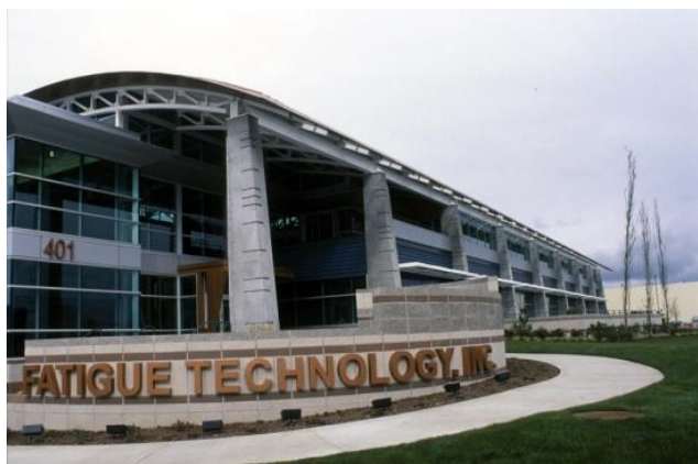
30. Existing light industrial/warehouse
