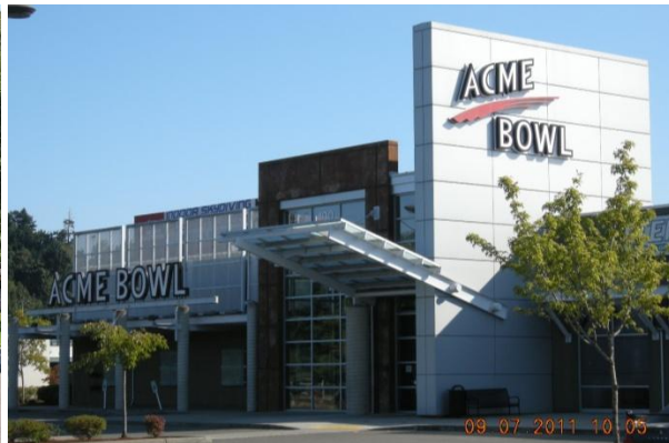
Acme Bowl – redevelopment of warehouse
