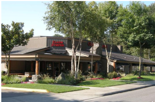
Claim Jumper – new construction built to the Corner of Southcenter Pkwy and 180 th Street
