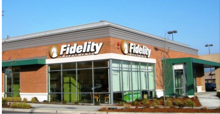
Pad building on Westfield Site built to the back of sidewalk on Strander
