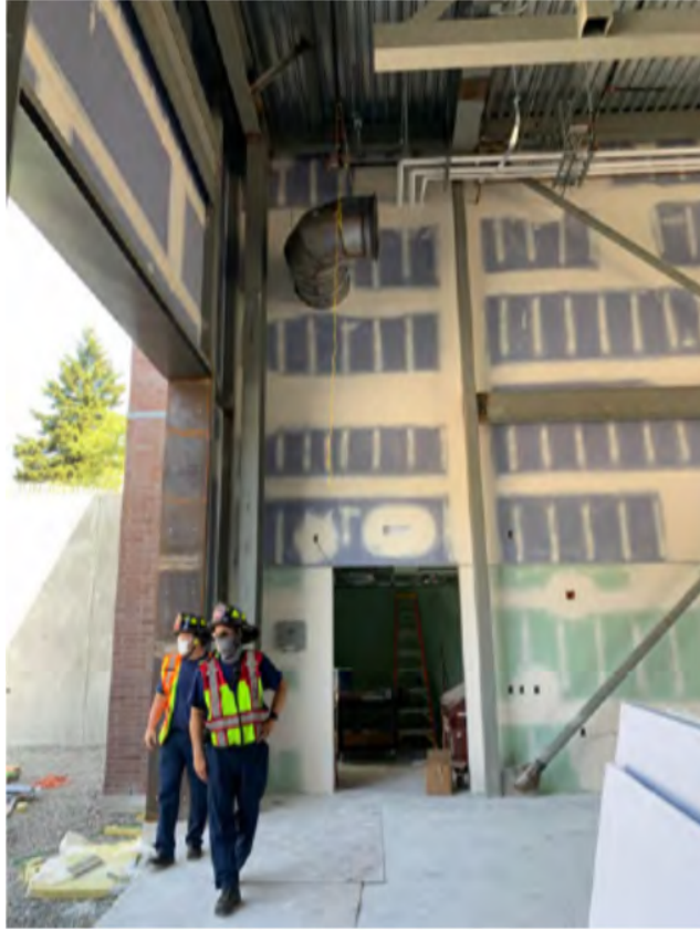
Nederman Ductwork being installed in the Apparatus Bay
