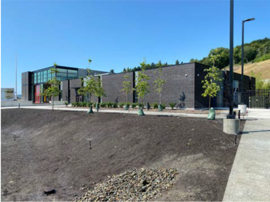
Trees in place at east façade with irrigation
