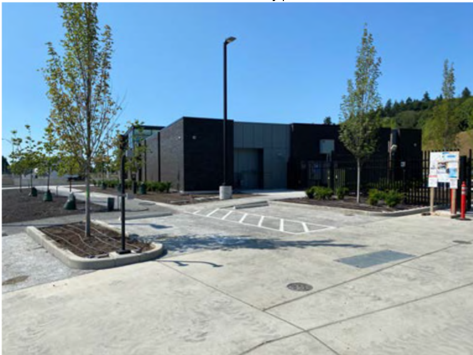
Trees installed at entry planters
