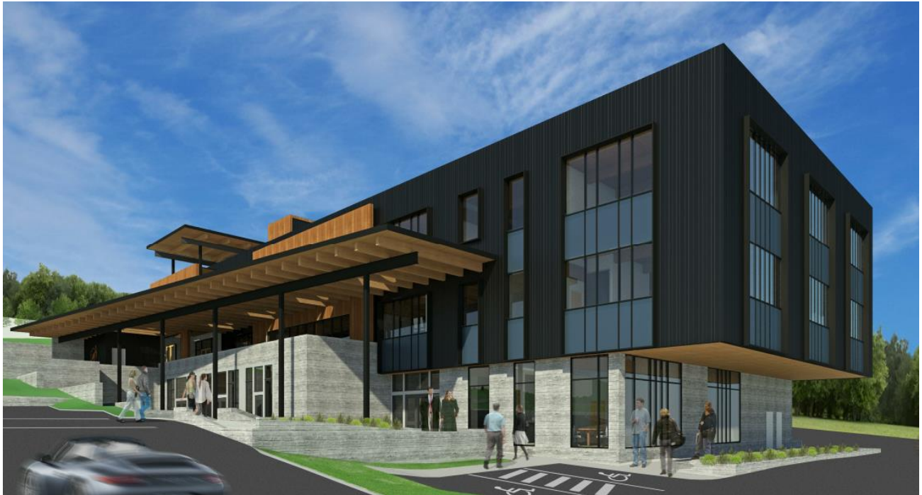
Fig. 14: Building rendering with canopy shown along southern elevation (left) and cantilevered second and third floors over eastern walkway (right).
