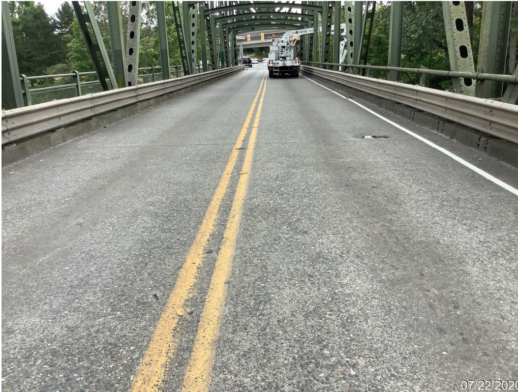
Inspection Photo 1 – Deck View Looking South
