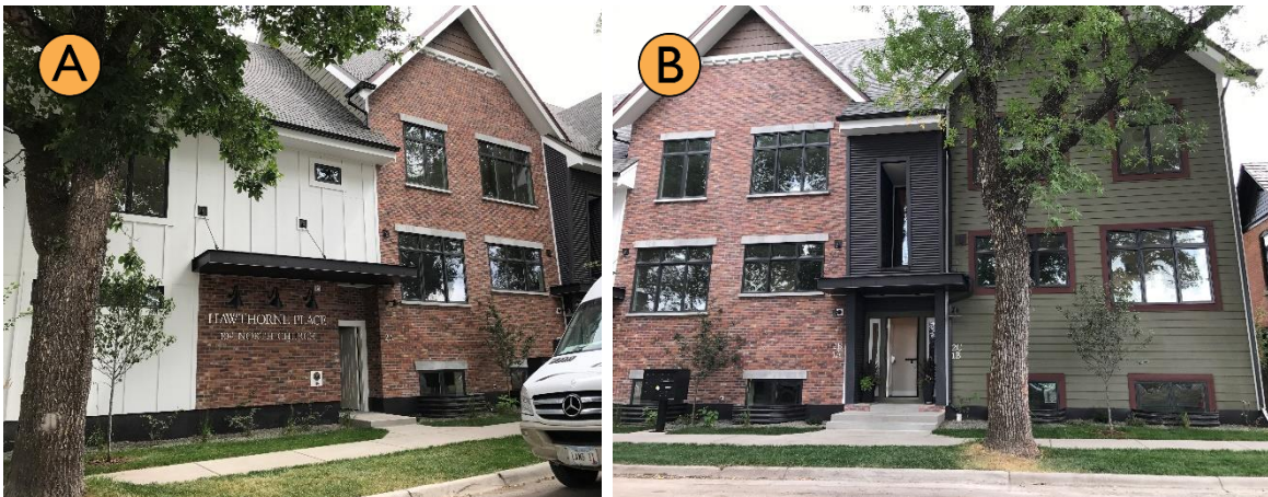
Figure 3.4.D Acceptable and unacceptable cementitious wall board examples.
