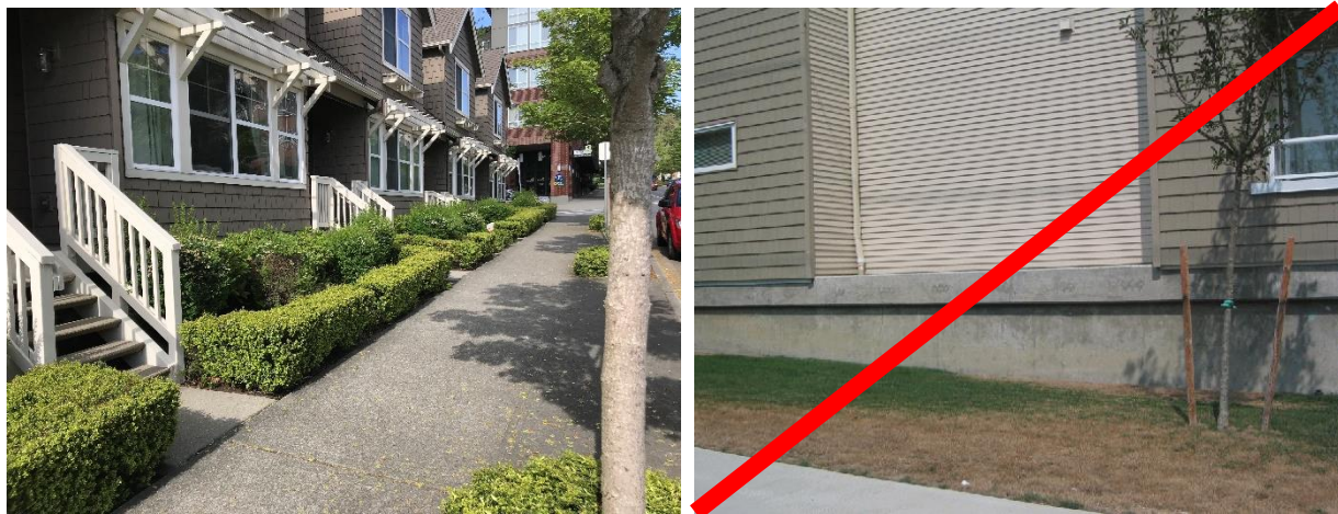
Left: Foundation with adequate landscape screening. Right: Foundation with inadequate landscape screening.
