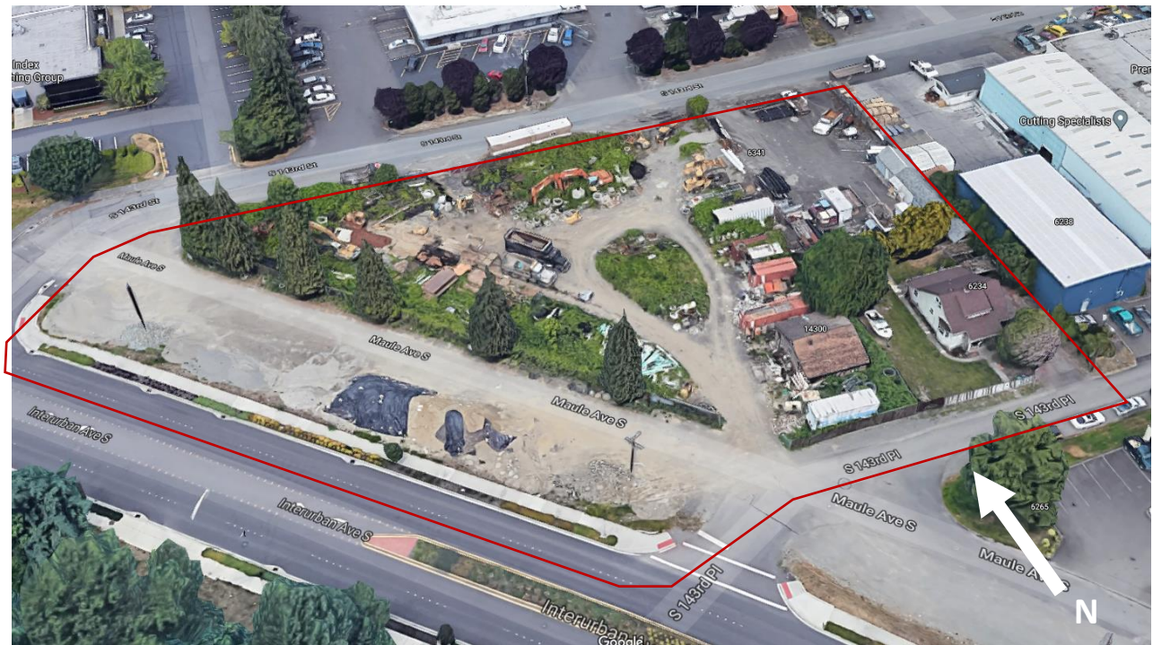
Fig. 3: Existing site conditions.
