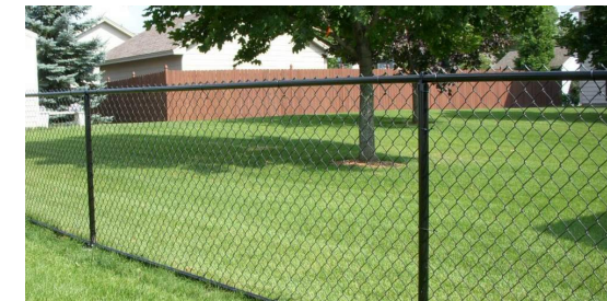
6' TALL VINYL COATED CHAIN LINK FENCING
