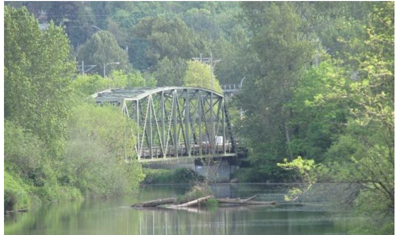
Existing 42nd Ave S Bridge
