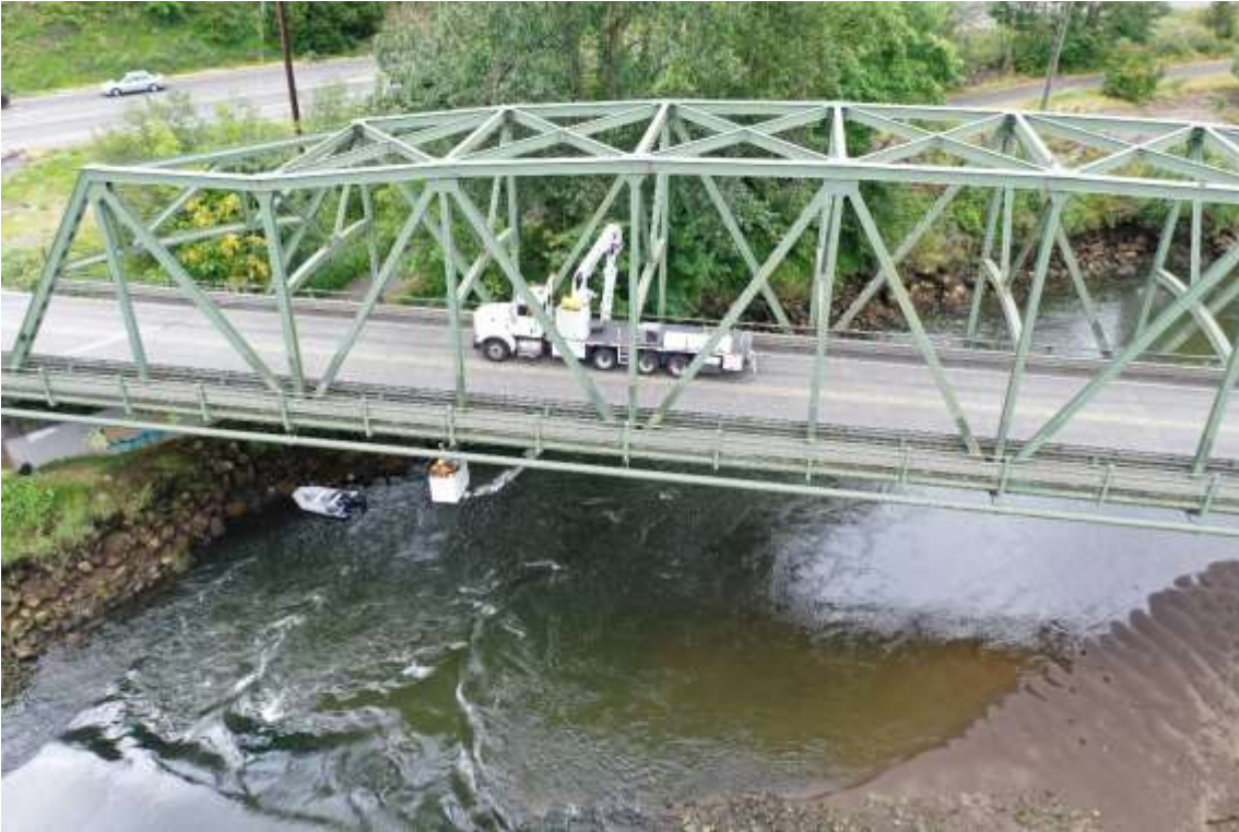
Photograph 1: Overall view of the in-depth inspection.
