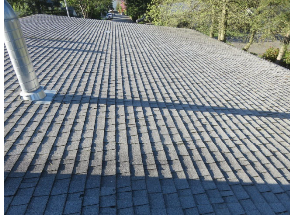
Upper Roof of the Building
