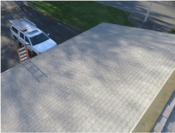
Lower Roof of the Building
