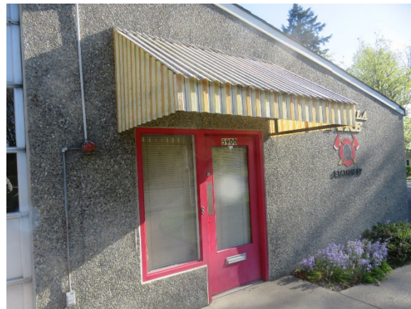
South Entrance to the Building
