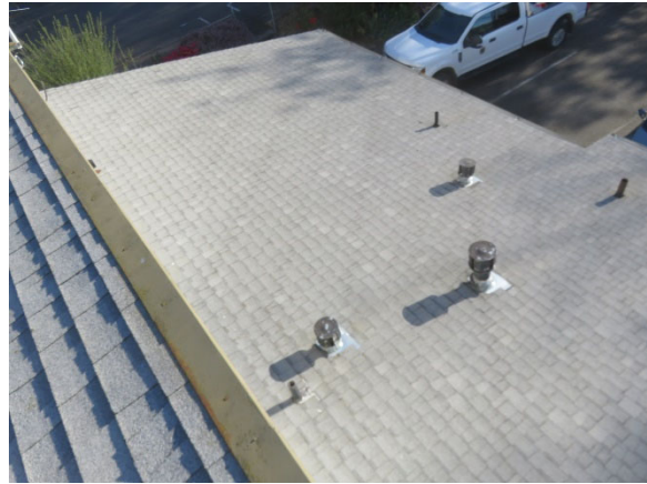
Lower Roof of the Building
