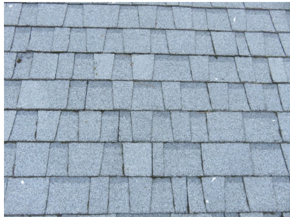
Close-up of Upper Roof of the Building
