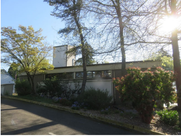
West Side of the Building
