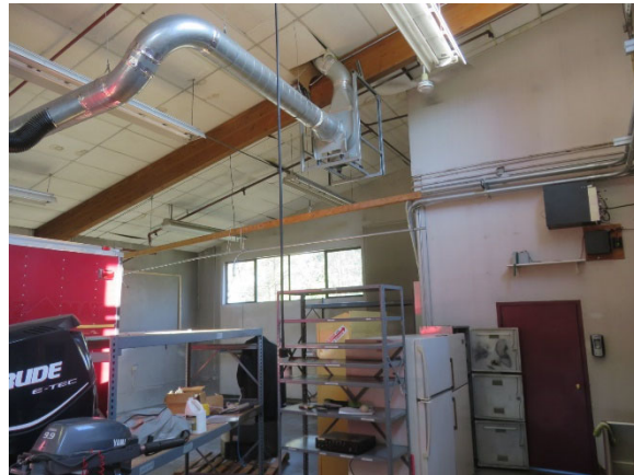
Glue-Laminated Beams Supporting the Roof
