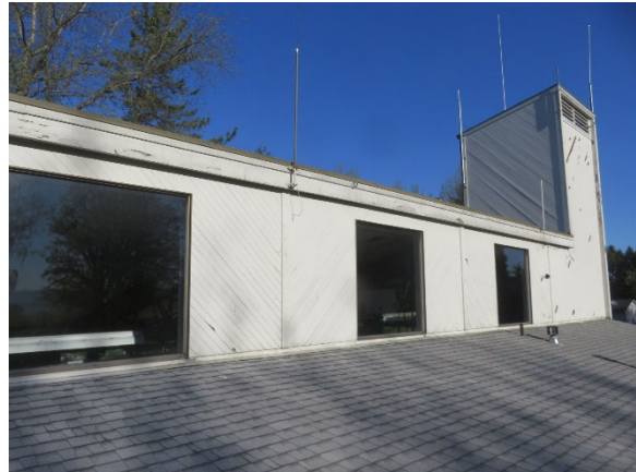
Clerestory at the East Side of the Building
