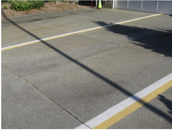
Concrete Parking Lot at the South Side of the Property
