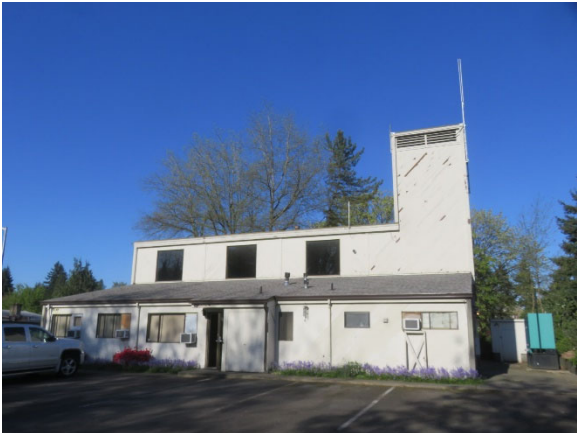
East Side of the Building
