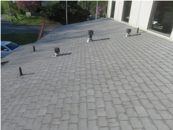
Lower Roof of the Building
