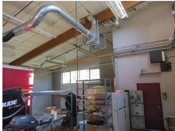
Glue-Laminated Beams Supporting the Roof
