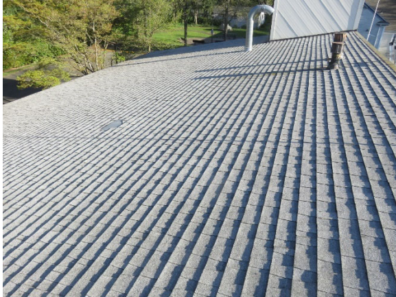
Upper Roof of the Building
