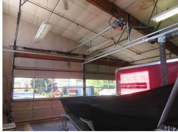
Engine Garage Bay
