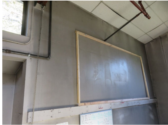
Concrete Wall Interior
