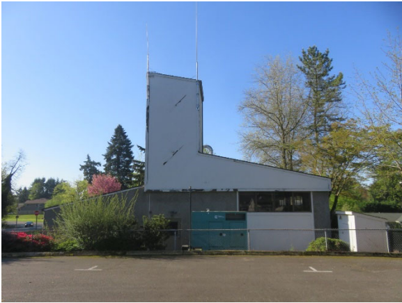
North Side of the Building
