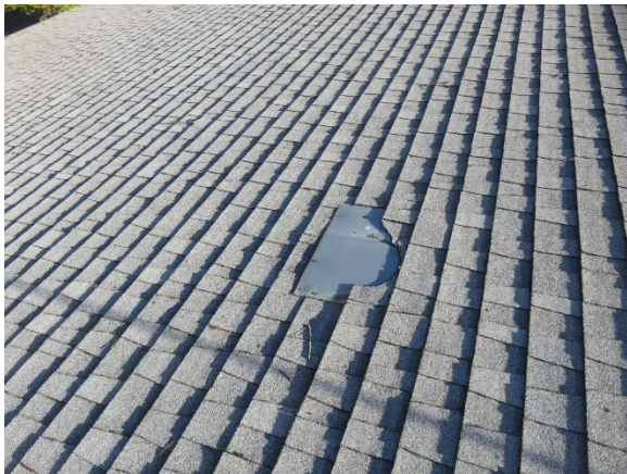
Repairs of Former Damage to the Upper Roof
