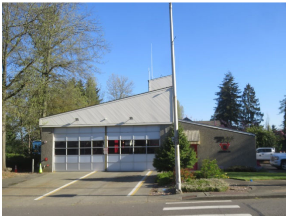
South Side of the Building
