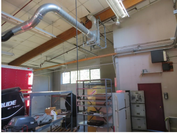
Engine Garage Bay
