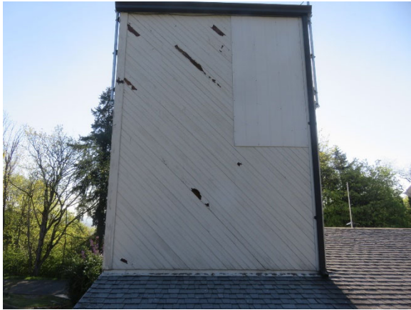
West Side of the Tower
