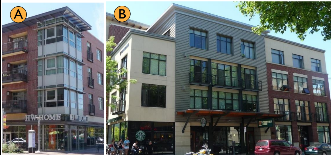
Figure 3.4.B Acceptable metal siding examples
