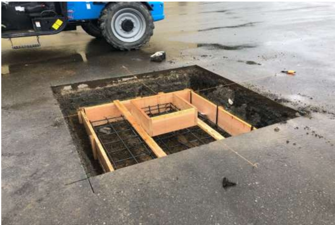
EXTERIOR FOOTING FORMS
