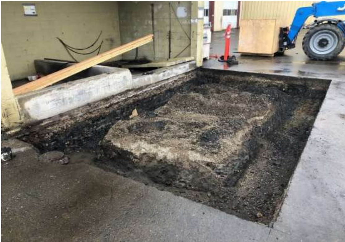
FOOTING EXCAVATION AT COMPRESSOR BUILDING
