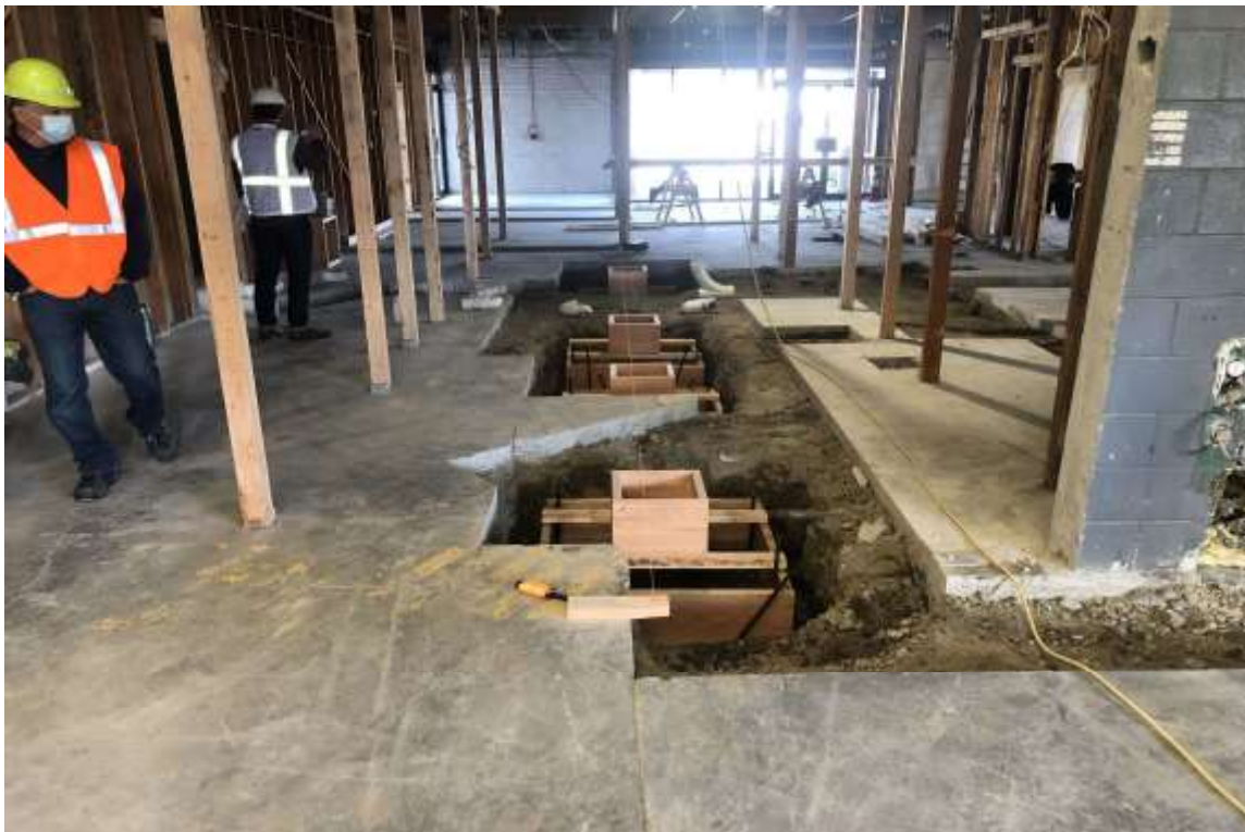
OFFICE AREA FOOTING FORMS IN PLACE
