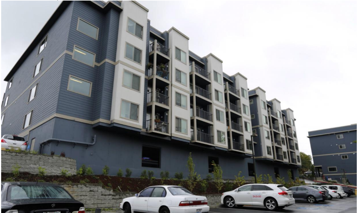
Figure 33. Example of a 4-over-1 Podium Development with Structured and Surface Parking Source: CoStar Location: Altitude Apartments, Renton, WA
