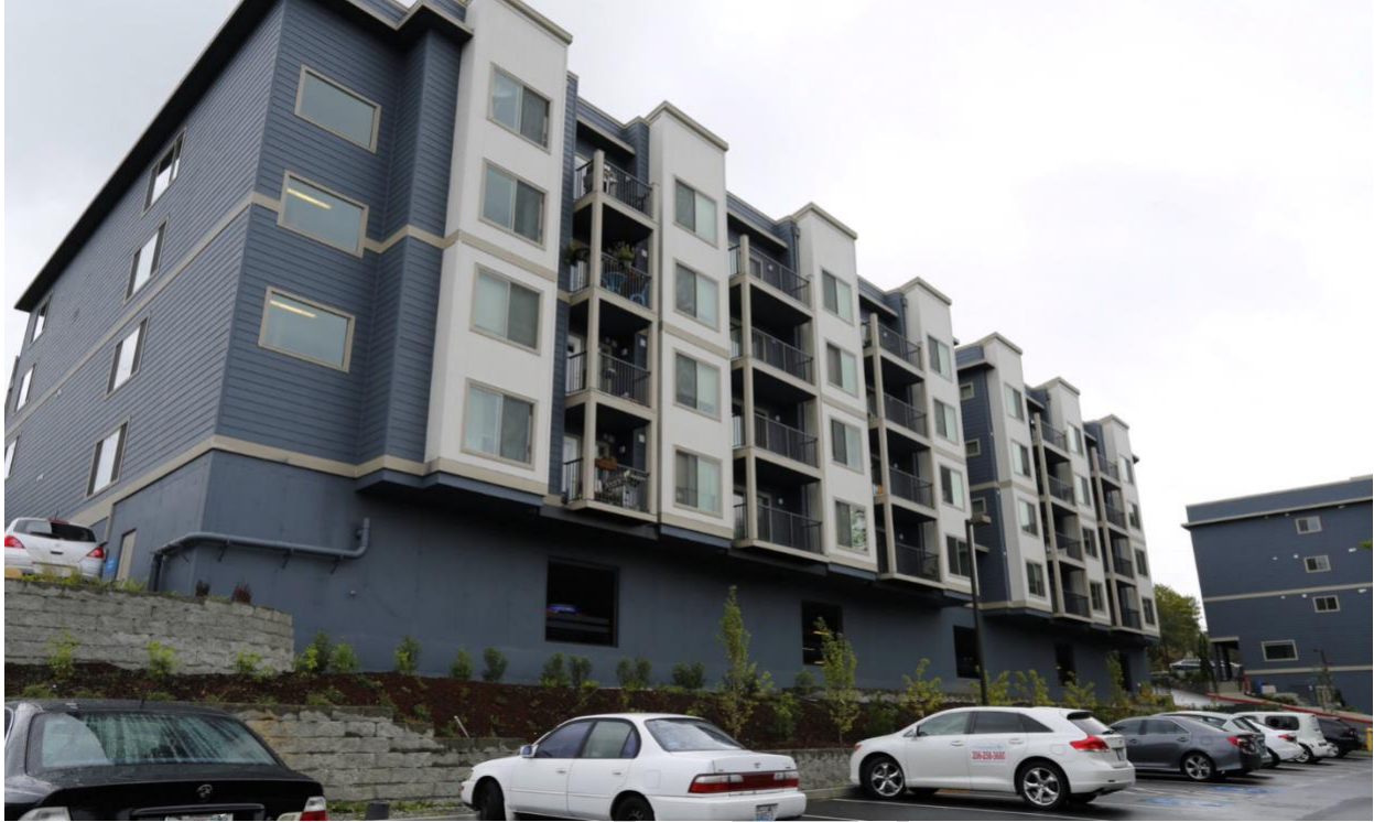
Figure 33. Example of a 4-over-1 Podium Development with Structured and Surface Parking Source: CoStar Location: Altitude Apartments, Renton, WA
