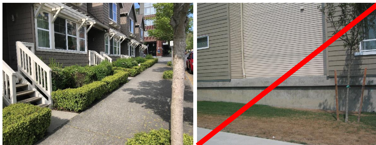
Left: Foundation with adequate landscape screening. Right: Foundation with inadequate landscape screening.
