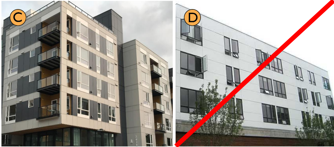
Figure 3.4.D Acceptable and unacceptable cementitious wall board examples.
