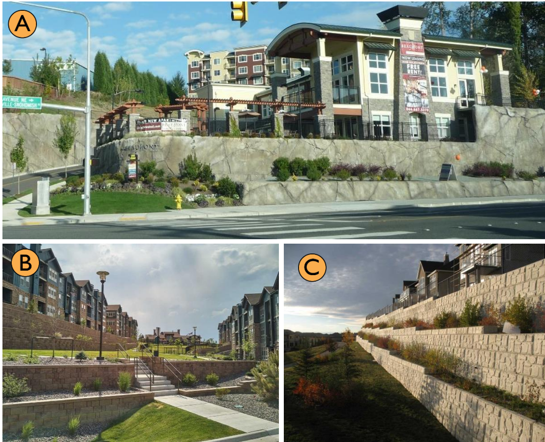
Figure 2.8.B Appropriate retaining wall terracing.
