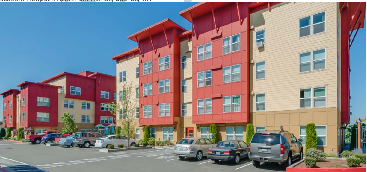
Figure 31. Example of a Wood Frame 4-Story Prototype
