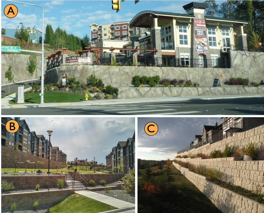
Figure 2.8.B Appropriate retaining wall terracing.
