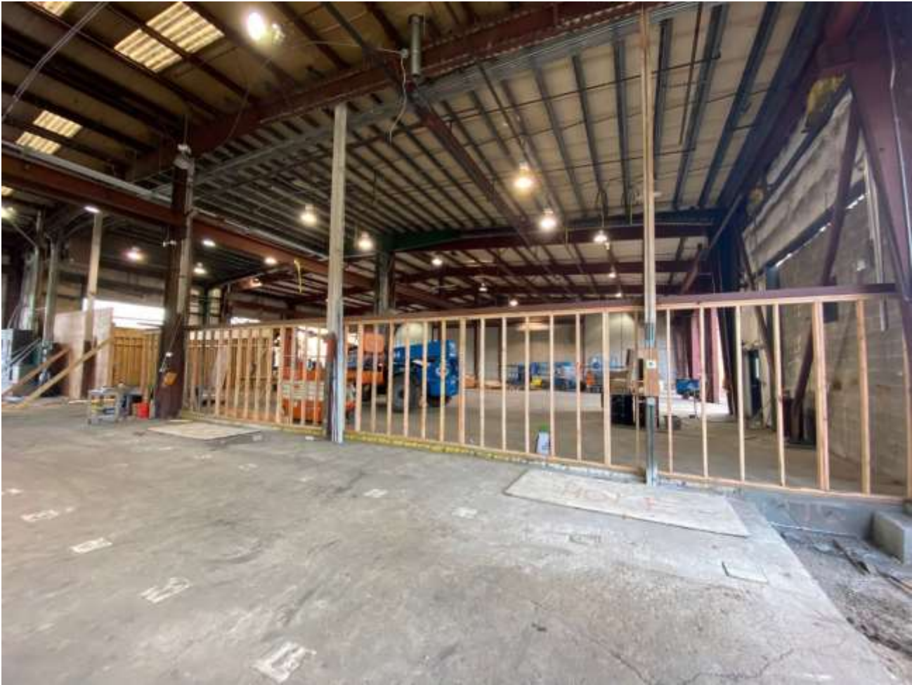
Framing in West Building
