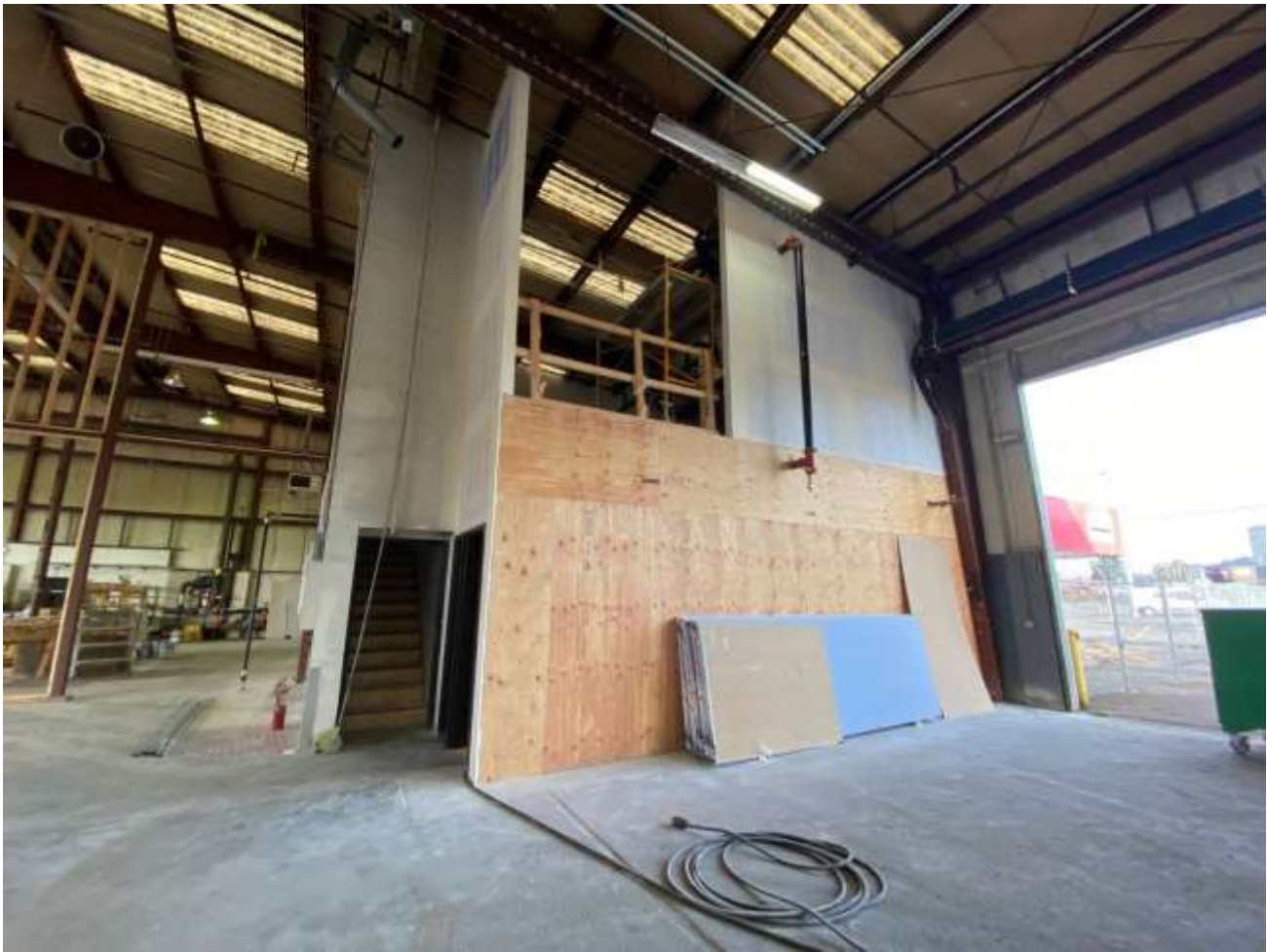
Office Space in Northwest Side of Building
