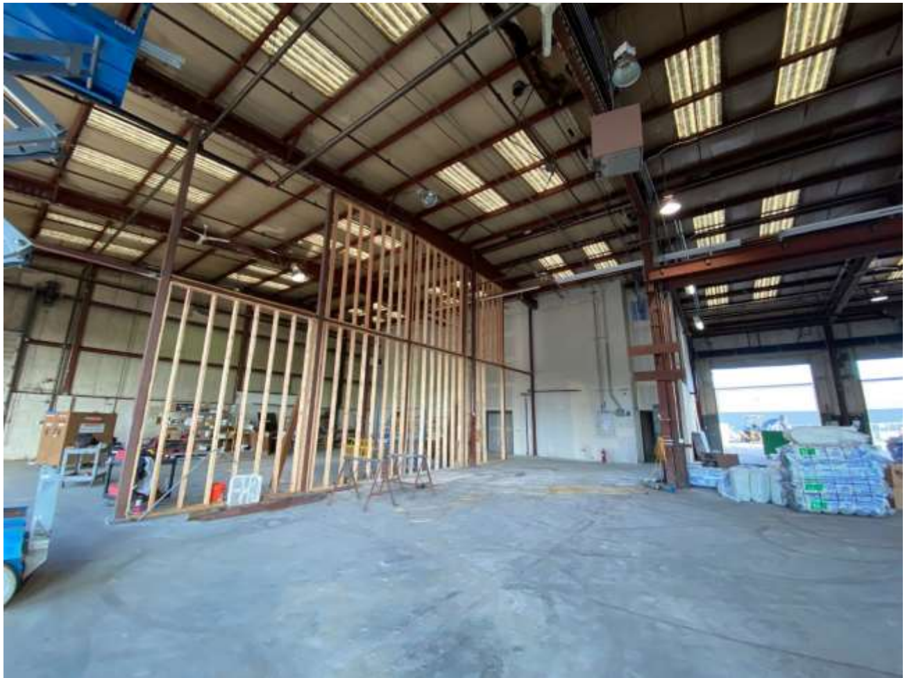
Framing in West Building
