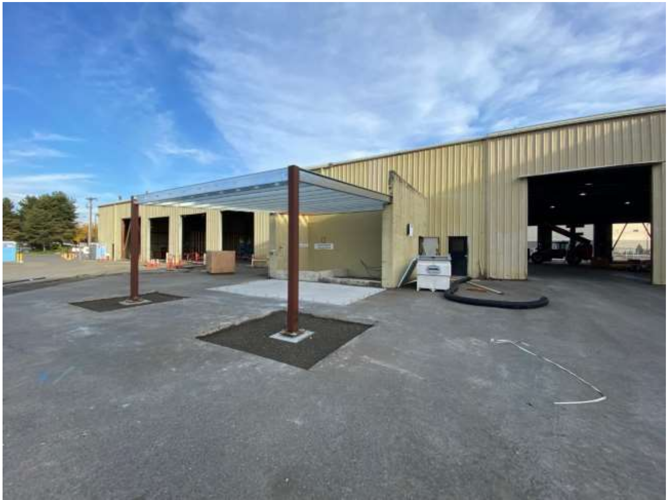
South Side of Building – Shed Roof
